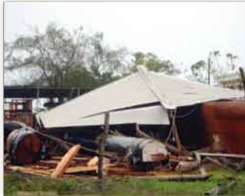
Photo 10: Destruction of dwelling houses by TC Rene, 2010, SNC Project, Tonga 2010.
