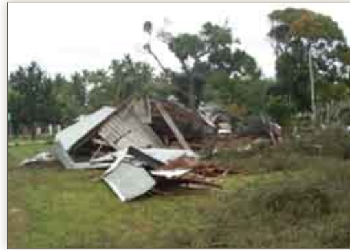
Photo 13: Tornadoes impacts on 'Utulau village, MoW, 2004.
