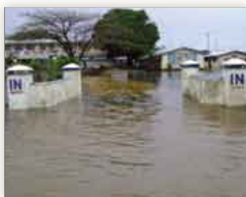
Photo 1: Flooding of St. Andrew's High School from heavy rainfall, 2009 SNC Project, MECC, Tonga.
