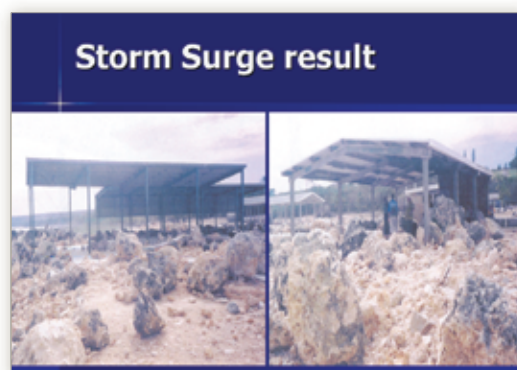
Photo12: Strong storm surge damaging Nafanua Harbour, MoW, 2003.
